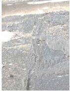
al 10 cm x 10 cm x 10 cm. patch on the lower right hand side part of the trench (Figure 2). The slab was cured using a heating blanket for 24 hours. A smaller second patch was also casted with a slightly modified geopolymer formulation.
